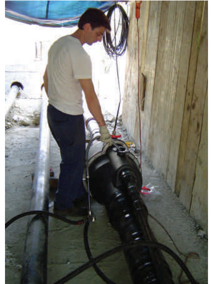
▲ Phoenix International's 2K Resin offers MV and HV underground joint protection
