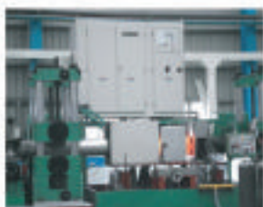
24" Pipe Mill And Annealing
