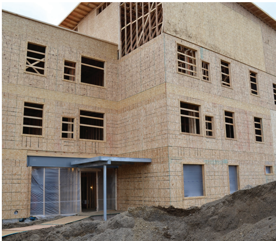
Construction is underway at the Gage East Apartments.
