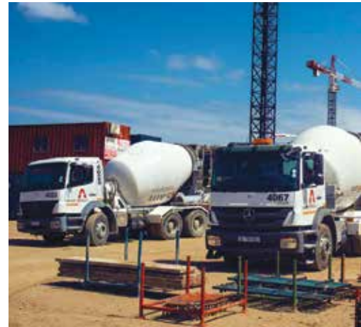
AfriSam delivers 600 m 3 of concrete to the site every day.
