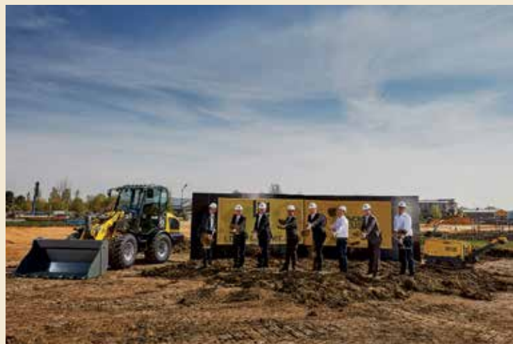
The silver-spade ceremony was held on 22 April and the first employees will be moving into the four-storey administration building and test hall by the end of the year.
