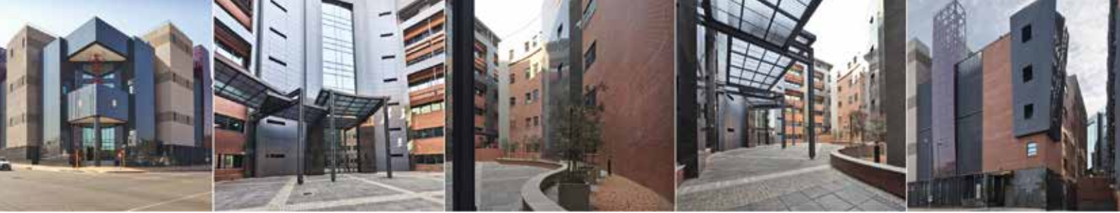
Limpopo High Court, a GVK-Siya Zama project completed in October 2015.
