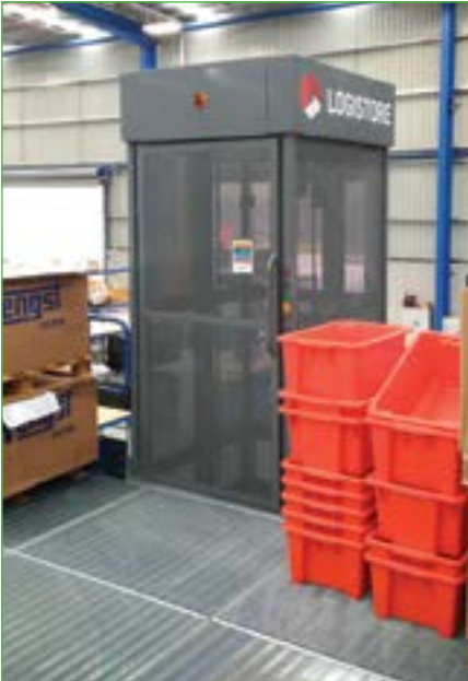
Logistore Goods Hoist upper level entrance
