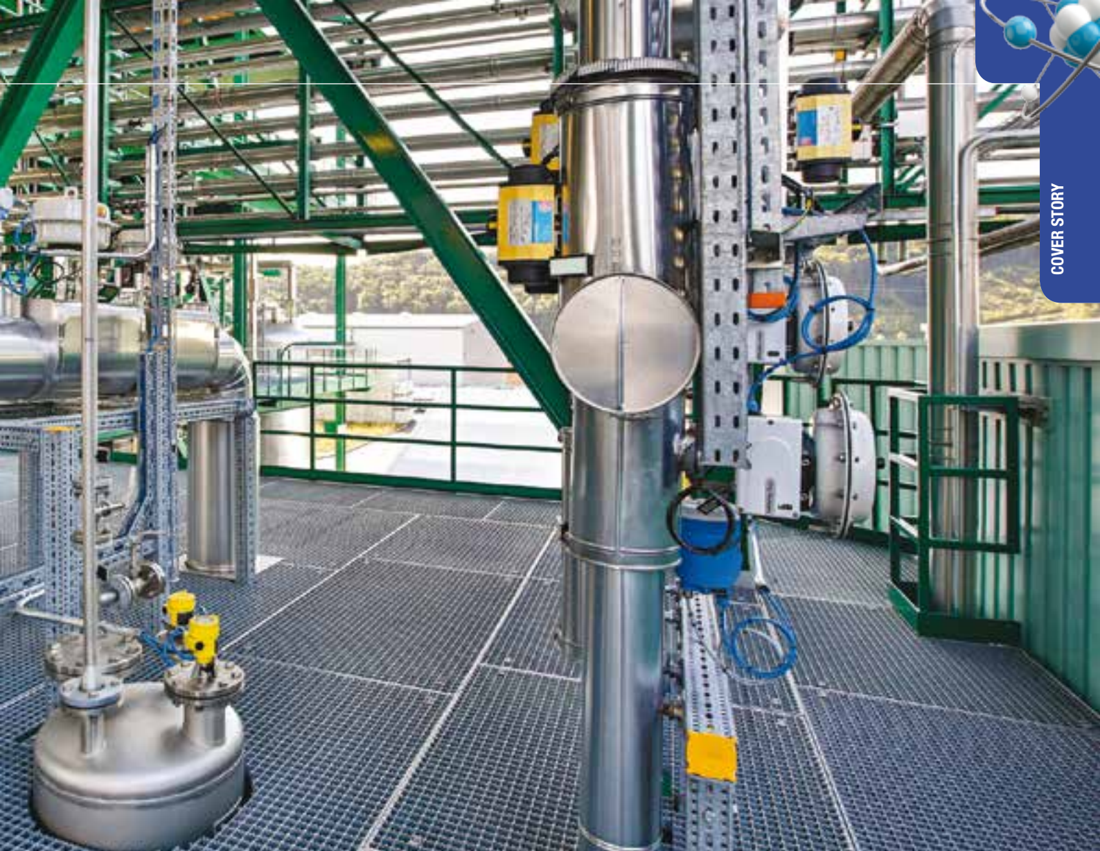
A radar beam with 80 GHz only reflects from the product surface. A 26 GHz beam also reflects signals from agitators and internal fixtures.
