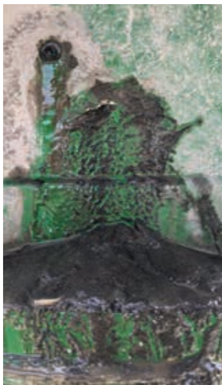
The weep hole allows inspection of the cyclone to be done while it is in operation.
