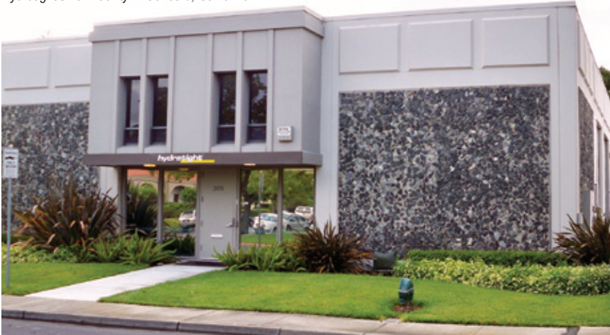
Hydratight's new facility in Concord, California
