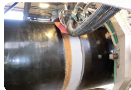
Field joint blast & coat
