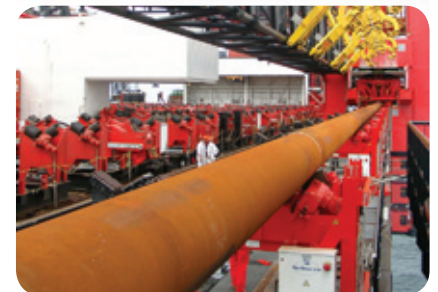
Offshore pipe handling
