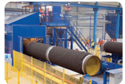
Concrete weight coating
