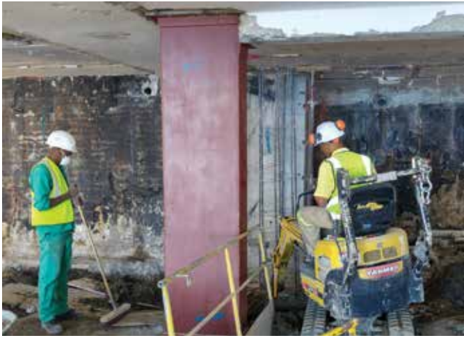
Internal excavations underway, with steel-clad pillar in the centre.
