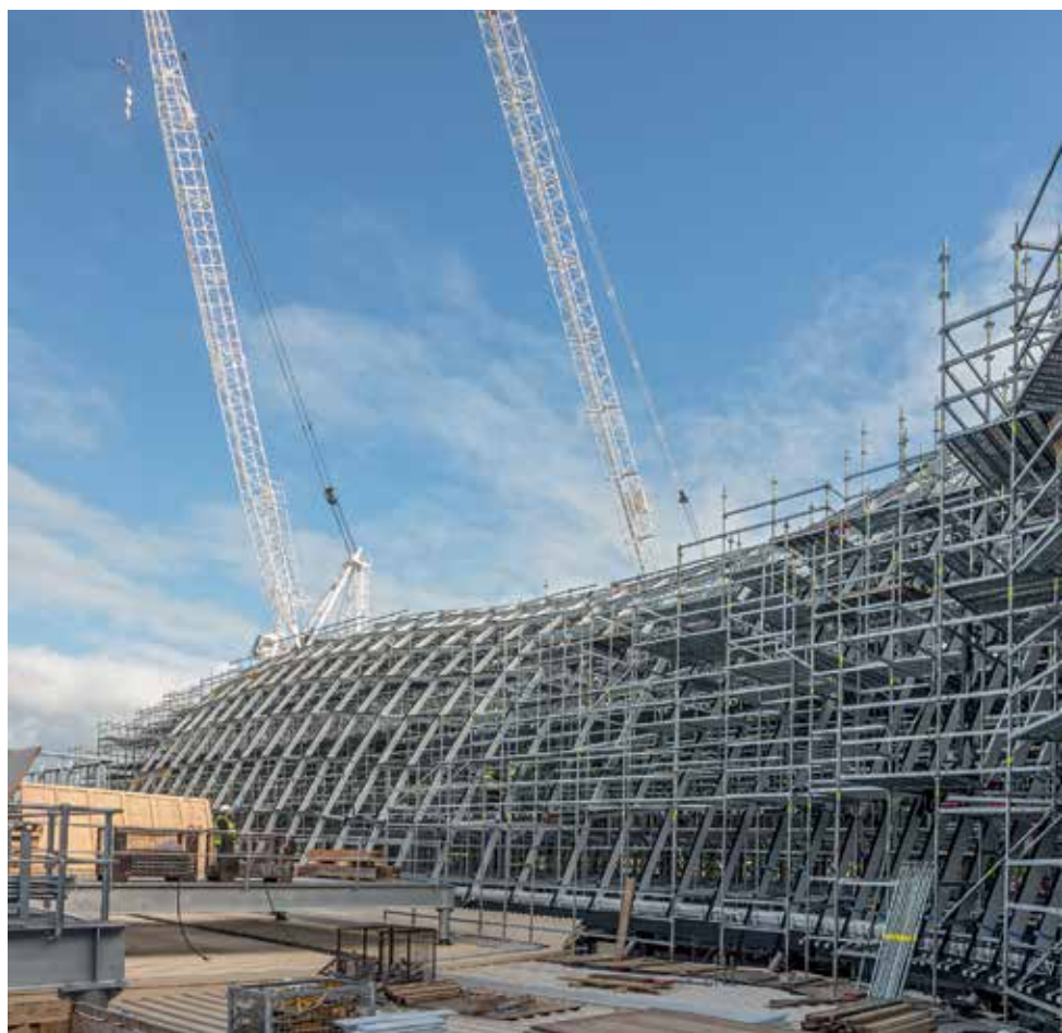
BELOW: The PERI UP Flex Modular Scaffolding was adapted to suit the complex-shaped glass roof structure: all working areas could be easily and safely reached while every load transfer was optimally planned.
