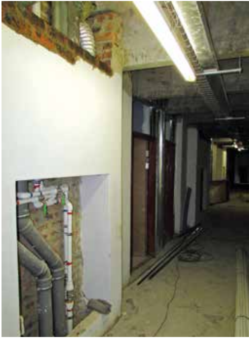
Precast wall units that have been tested at the manufacturer's facility are crucial to the acoustic requirements of the interior walls.
