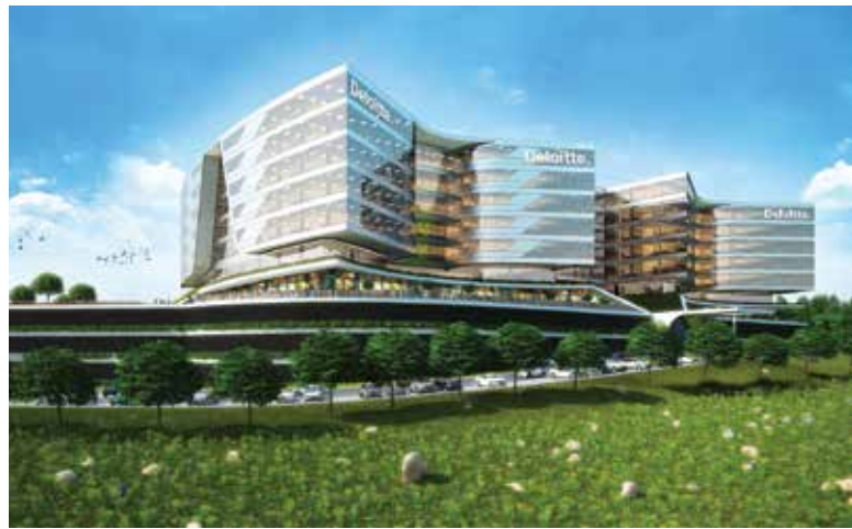
Opening in 2020 is Deloitte's new Gauteng head quarter building which has a price tag of more than R1-billion.
