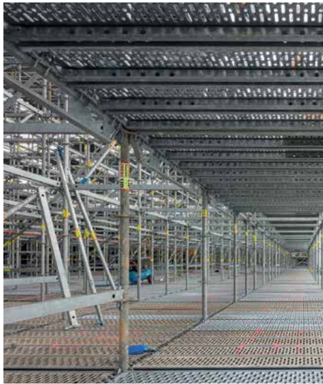
BOTH PHOTOS: All working levels could be completely covered with PERI UP Flex while the flat and even work areas were free of any tripping hazards. (All Photos: PERI GmbH)
