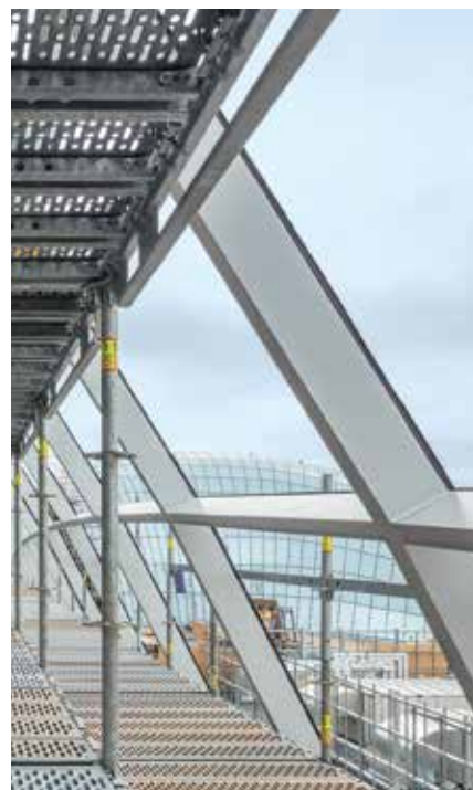
BOTH PHOTOS: All working levels could be completely covered with PERI UP Flex while the flat and even work areas were free of any tripping hazards. (All Photos: PERI GmbH)
