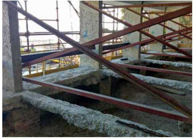
Steel braces provide support while this apartment's floor is deepened.
