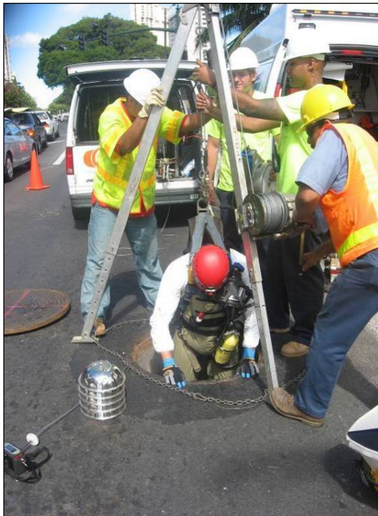
Photo 1. Confined Space Entry
