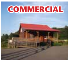
61377 - FANCY GAP - LOG CABIN, 2 BR, 1 BA, 1608 SF, PARTIAL FINISHED BASEMENT W KITCHEN, PORCH. $159,000
