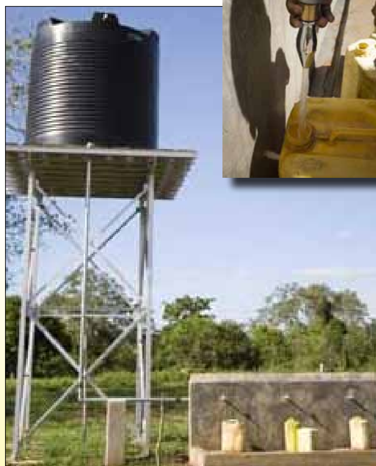
A typical 3-point water supply, Kamuli District Inset: A self-closing water tap prevents wastage
