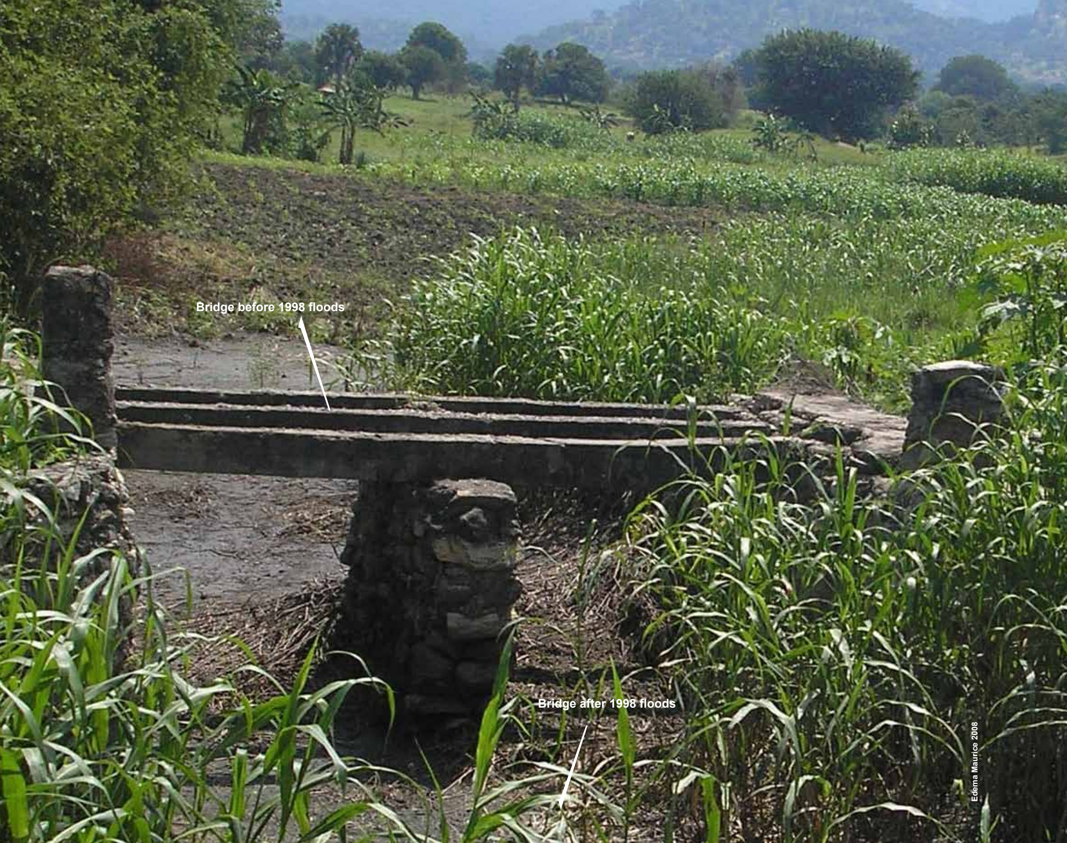
Shifted bridge as result of flooding on Ebemi stream along the Laropi-Dufile Road
