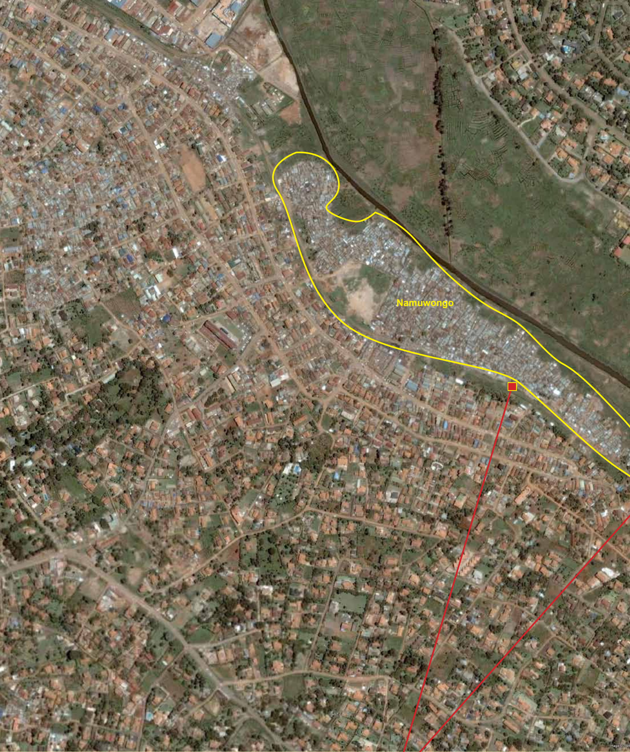
Construction of houses in Nakivubo wetland, Kampala (2007)
