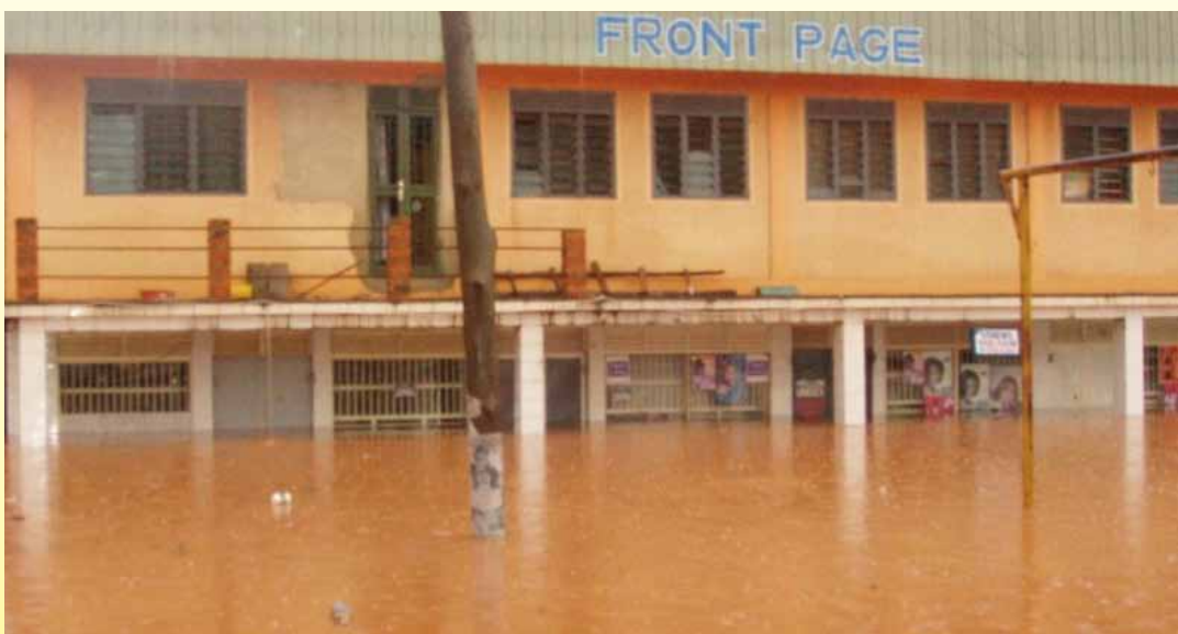
These buildings were constructed in wetlands which are the water ways for drainage into Lake Victoria. The houses were flooded in 2007 temporarily interfering with traffic and business along the Kampala-Entebbe highway.
