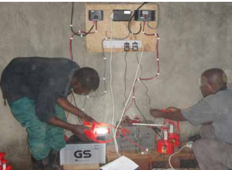
Solar energy: phone, battery and lantern charging at Wobutungulu by Joint Energy and Environment Projects (JEEP)
