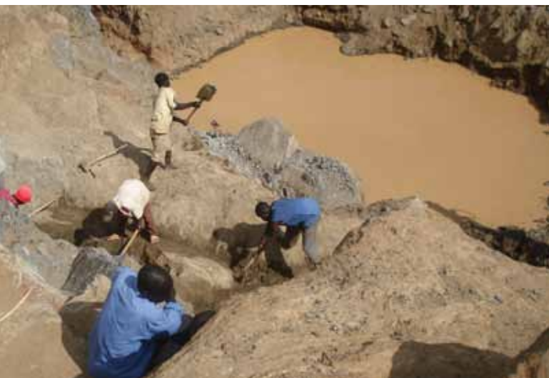
Construction of Nyagak Hydro electric power plant
