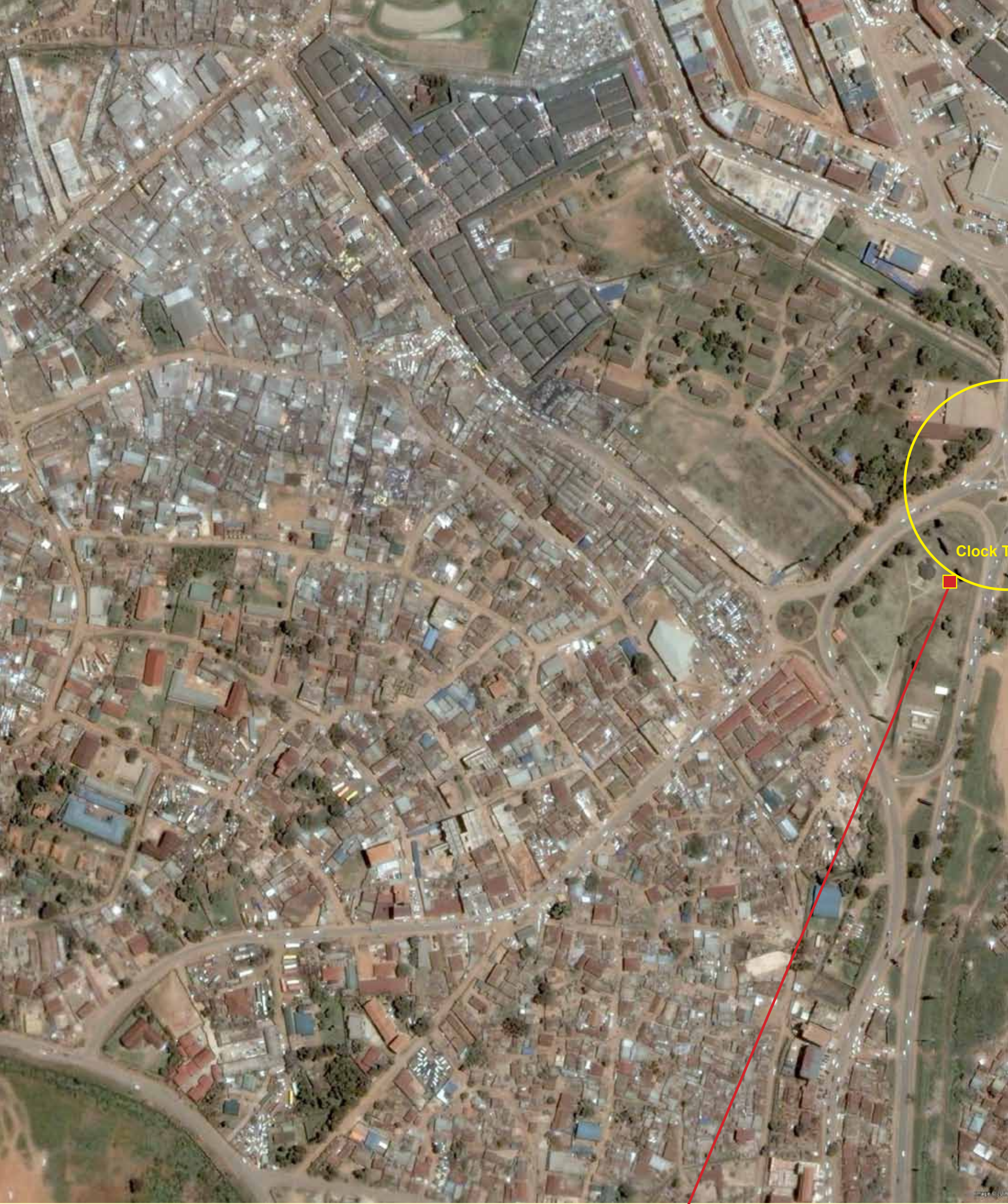
Flood prone area at Clock Tower junction, Kampala (2009)
