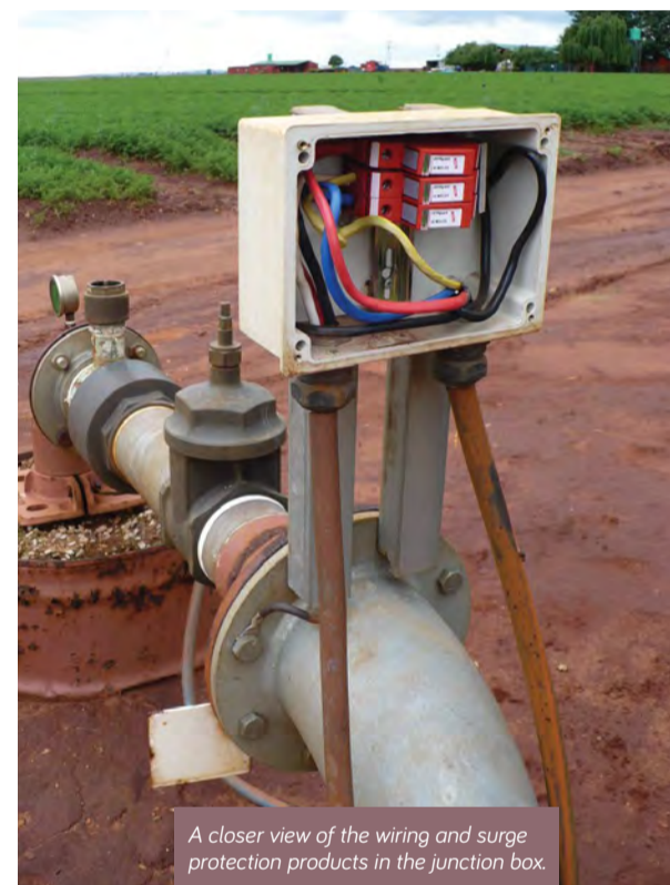
A borehole outlet pipe being fitted with earthing and surge protection units housed in the junction box.
