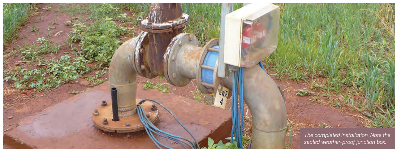
A borehole outlet pipe being fitted with earthing and surge protection units housed in the junction box.
