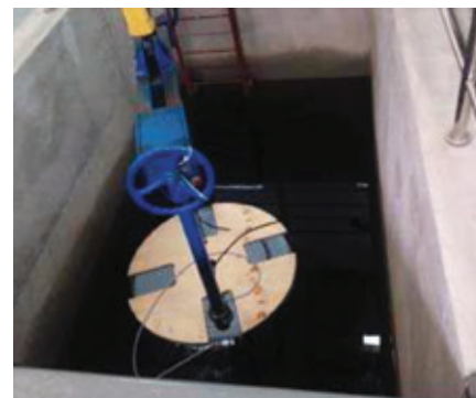
▲ Figure 1: Micro-duct with cable soaked in water
