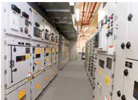
LV and MV Switchboards inside E-House
