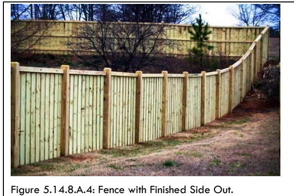
Figure 5.14.8.A.4: Fence with Finished Side Out.
