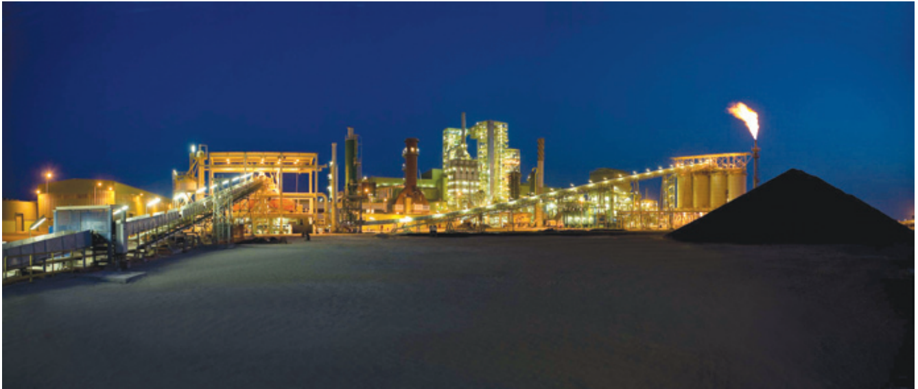
▲ Emirates Steel 1.6 million tpy HYL Energiron plant with HYTEMP System, Abu Dhabi
