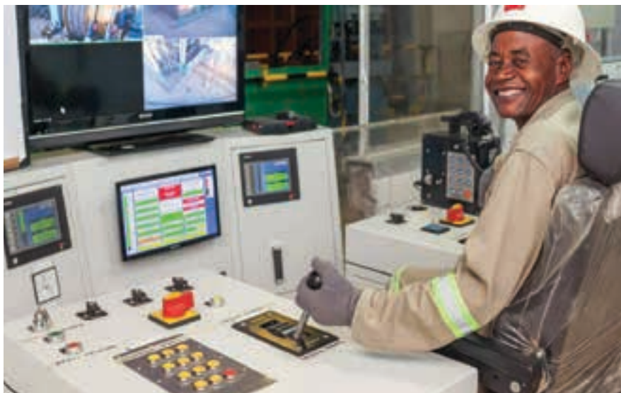
Control room operator at Kipushi's Shaft 5 (photo: Ivanhoe).
