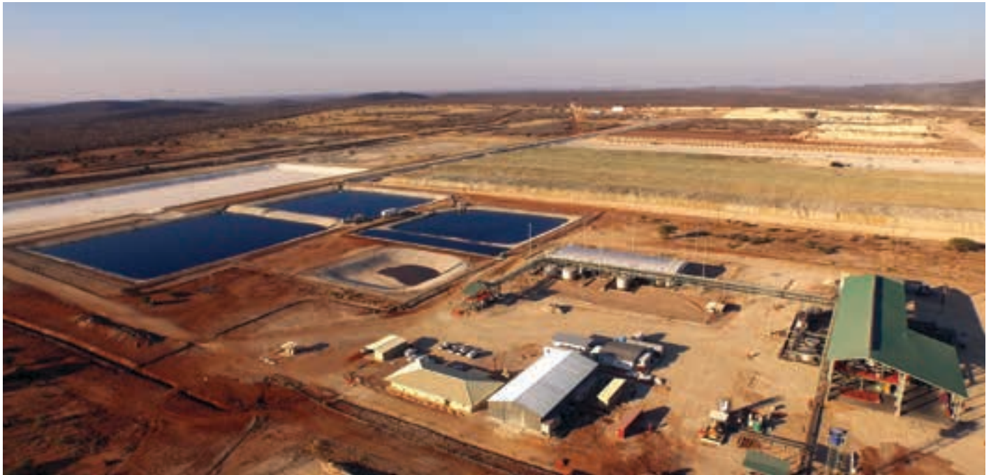
The Tschudi open-pit, heap leach, SX-EW operation near Tsumeb in northern Namibia. Its current capacity is 17 kt/a of LME Grade A copper cathode (photo: Weatherly International).
