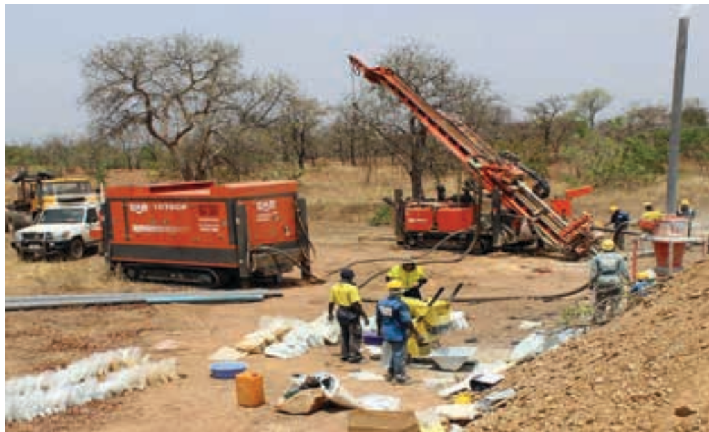
Drilling at the Namdini project in northern Ghana (photo: Cardinal).
