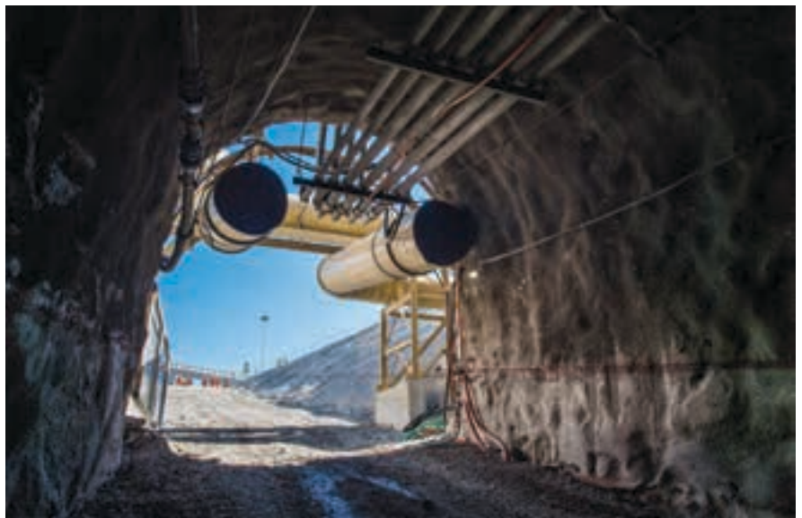
The portal to the Venetia Underground decline.
