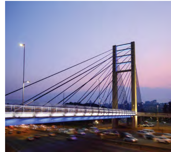
BEKA Schröder LED luminaires illuminate this iconic new bridge in Johannesburg
