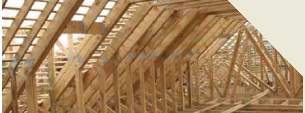
Prefabricated timber roof trusses
