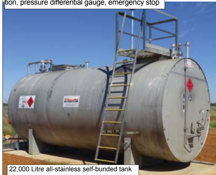
Tank inflill and dispensing pumps. Fitted with filtration, pressure differential gauge, emergency stop
