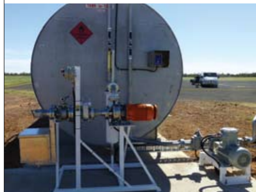
Tank inflill and dispensing pumps. Fitted with filtration, pressure differential gauge, emergency stop
