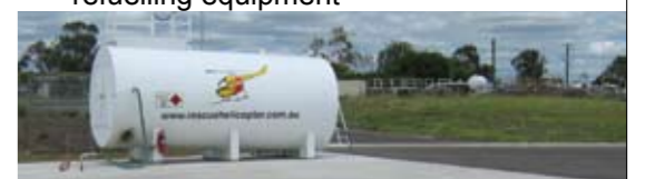
Self-bunded storage tank with on-demand pump system and emergency backup refuelling equipment
