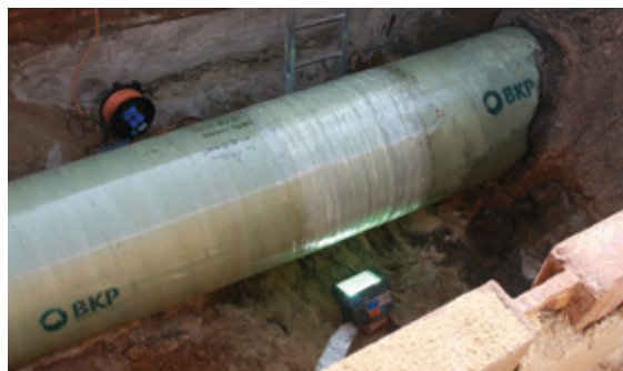
Curing of the GRP surface protection
