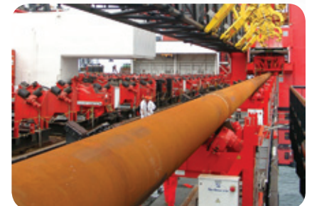
Offshore pipe handling
