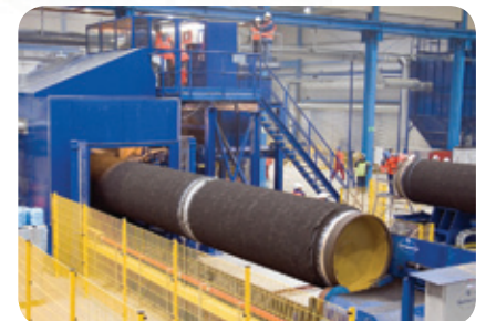
Concrete weight coating
