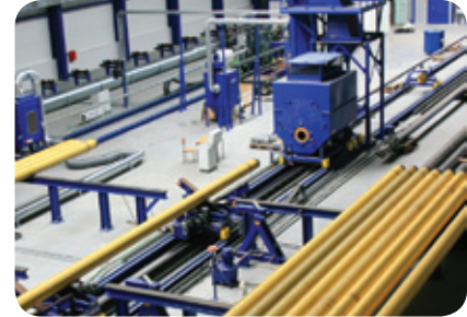
Internal blasting & lining
