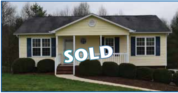
MLS# 881226 177 WESTBRIDGE PLACE, MT. AIRY - Ranch style home in Woodbridge Subdivision. 3BR, 2 full bath, full basement, nice large lot, deck, all appliances stay. New roof. Ready to move in..... $138,500
