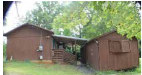
850932 - 202 ANNA BRYANT TRL - Wood floors and other materials were cut from the surrounding land. House has open kitchen, living area, dining area 1.5 BA, 2 BR and a detached screened in porch with storage on one end. HVAC system consist of individual Global Ductless Air Conditioner units in various locations throughout the house for a nice even heating and cooling. $67,900
