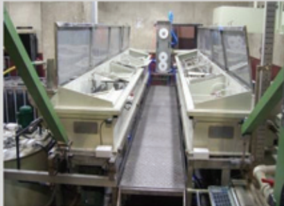
Electrolytic tinning plant (waste water free)
