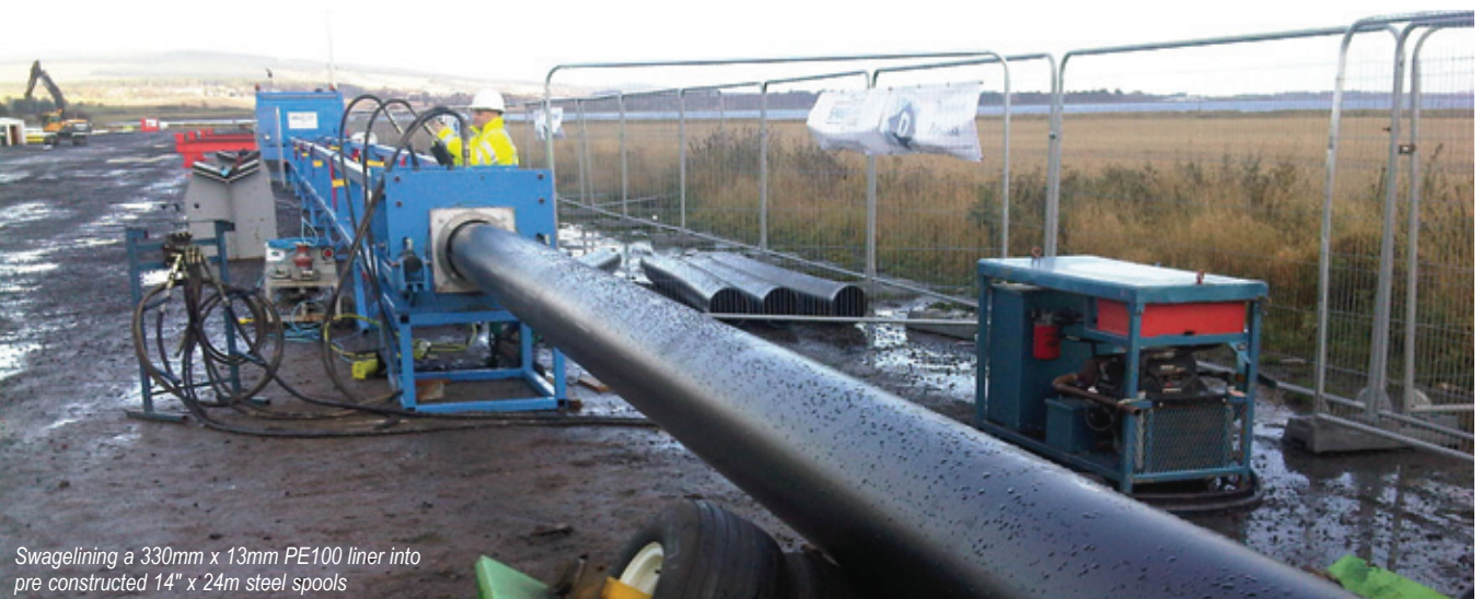
Liner Installation through the Weldlink connector
