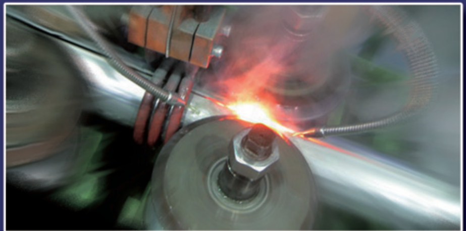
Automatic Stainless Pipe Welding Scene
