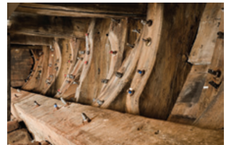
(Above) Over 5,000 bolts were positioned in Vasa after the ship was salvaged 1961. They were all fixed in the ship's existing bolt holes, where the original bolts had rusted through
