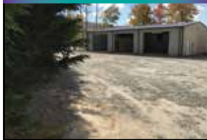
40'X60' (3) bay workshop/storage building just outside of Mount Airy. Excellent condition with (3) 10'X12' power lift overhead doors, full power, water stations, exhaust fan, floor drains, plumbed for bathroom, office space and more. $1800/month
