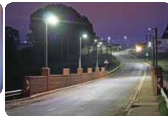
The lighting installation in Stutterheim that put the South African town on the international lighting map.
