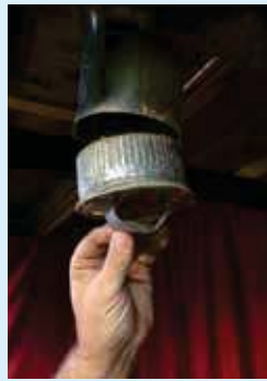
(above) Manual Lint Trap found in some ductwork. This should be cleaned.
