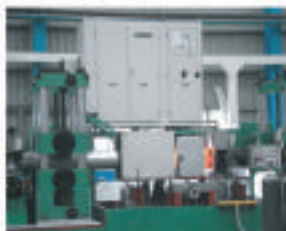
24" Pipe Mill And Annealing
