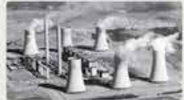
Lethabo Power Station
