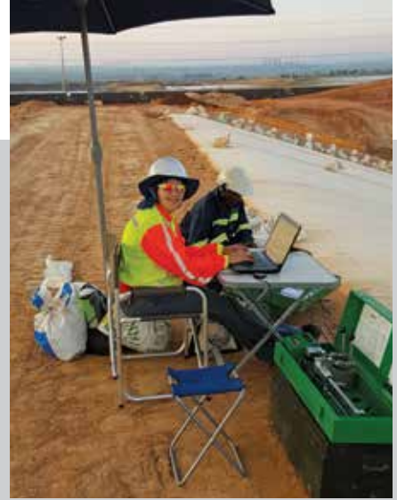
Capturing real-time data on site during the installation process.
