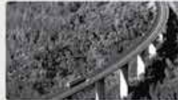
Hugo's River Viaduct
