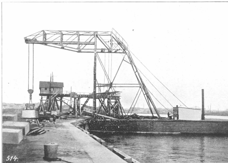
30 Tons Goliath Kran, Libau
