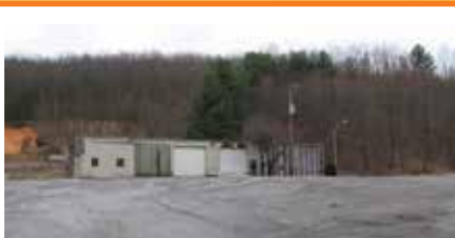
1500 Pump Hollow - Shop with 5 bay doors for the mechanic or business to be able to service your own equipment with additional open equipment shed offering 2 open acres along with 5 wooded acres joining Big Survey. $165,000
