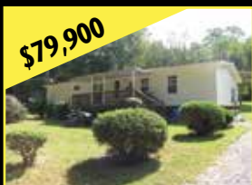
$79,900 MLS# 57582 - SPEEDWELL - 2 BR, 1 BA Ranch Home on an acre of land. Large laundry room. Covered front porch and outbuilding, fenced garden and plenty of privacy for one level living.
