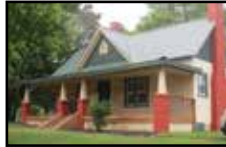
794628 - Renovated in 2014, 1,622 SF comm. bldg w/ street exposure of 10,000 vehicles/day on N. Bridge St., Elkin. New heat pump, wiring, windows, roof. $88.16 SF or $143,000
