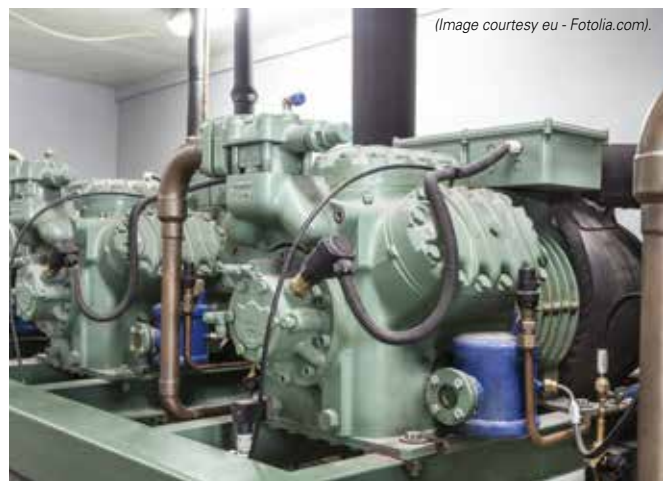
Figure 4: Monitoring of the gear lubrication in generator sets.
