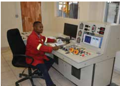
100 MVA 132 kV Testing Bay
