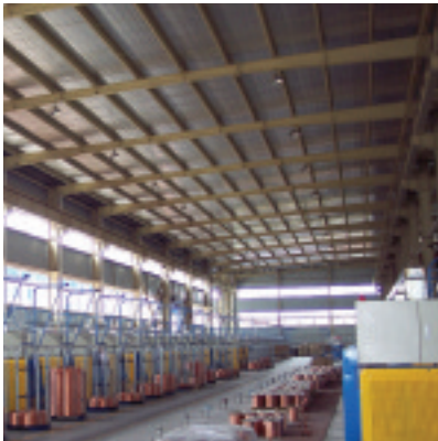
○ Wire drawing lines from Guanbiao Electrical Machinery Co Ltd
