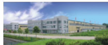
○ The Anhui Changjiang Jinggong Wire & Cable Machinery factory
