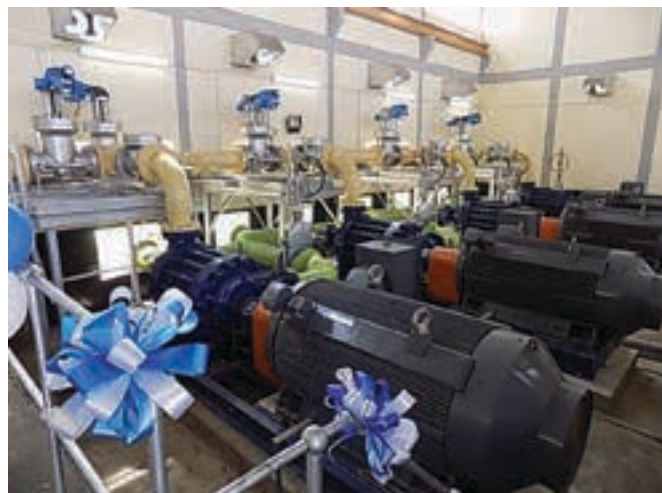
APE Pumps installed Mather+Platt pumps at the refurbished high-lift pump station at Chileka, Malawi. Eight PJ250H Mather+Platt multi-stage pumps capable of sustaining flow rates of between 750 and 900 m 3 /h and a maximum heads of 550 m were manufactured at the company's Wadeville facilities in South Africa.
