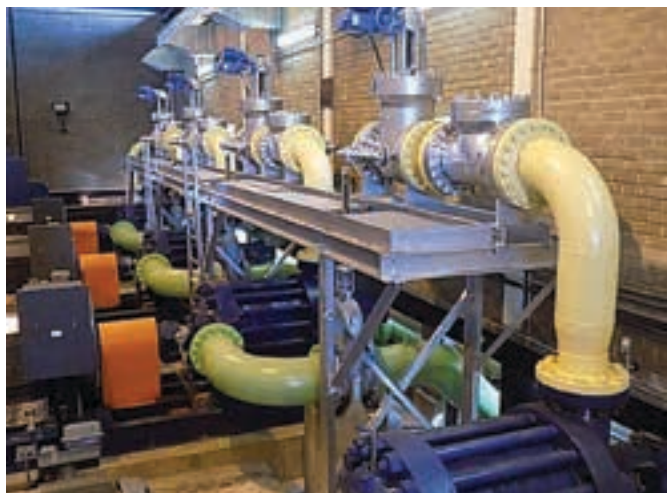
APE Pumps installed Mather+Platt pumps at the refurbished high-lift pump station at Chileka, Malawi. Eight PJ250H Mather+Platt multi-stage pumps capable of sustaining flow rates of between 750 and 900 m 3 /h and a maximum heads of 550 m were manufactured at the company's Wadeville facilities in South Africa.
