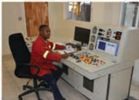
100 MVA 132 kV Testing Bay
