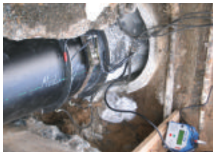
▲ The Simofuse technology integrated within the pipe modules can be operated with standard electrofusion welding machines
