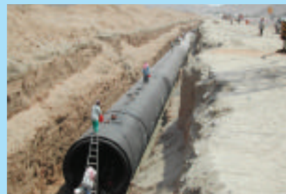
▲ Installation of 2,500mm diameter T-Lock lined pipes
