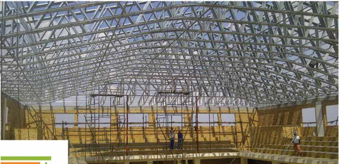
Clear span roof structure of 26m – Old Apostolic Church, Mayfield, JHB
