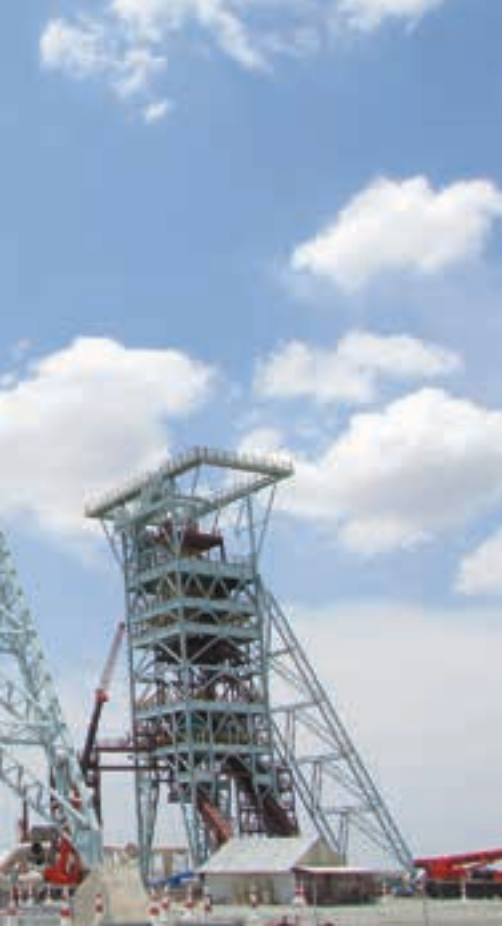
Above: The vertical shaft mucker (VSM): The use of VSM systems with clamshell muckers at Venetia is a South African first.
