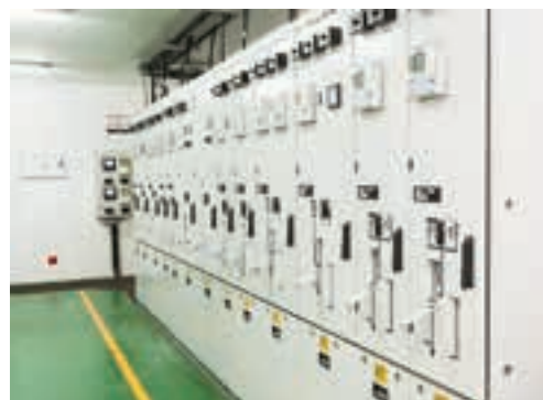
A typical medium voltage ABB gas insulated switchgear installation.
