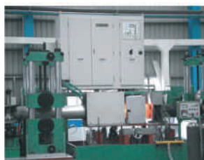
24" Pipe Mill And Annealing
