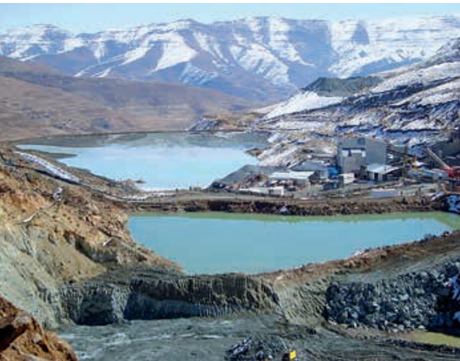
Liqobong in winter. This photo, taken in 2012, shows the original plant at the site which has now been removed.
