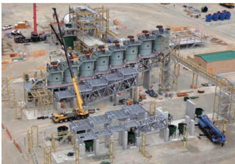
Flotation circuit construction at the WBJV Project 1 site.
