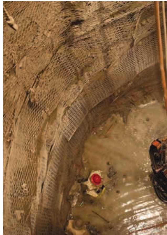
Looking up the ventilation shaft from the kibble towards the sinking stage (photo: Arthur Tassell).
