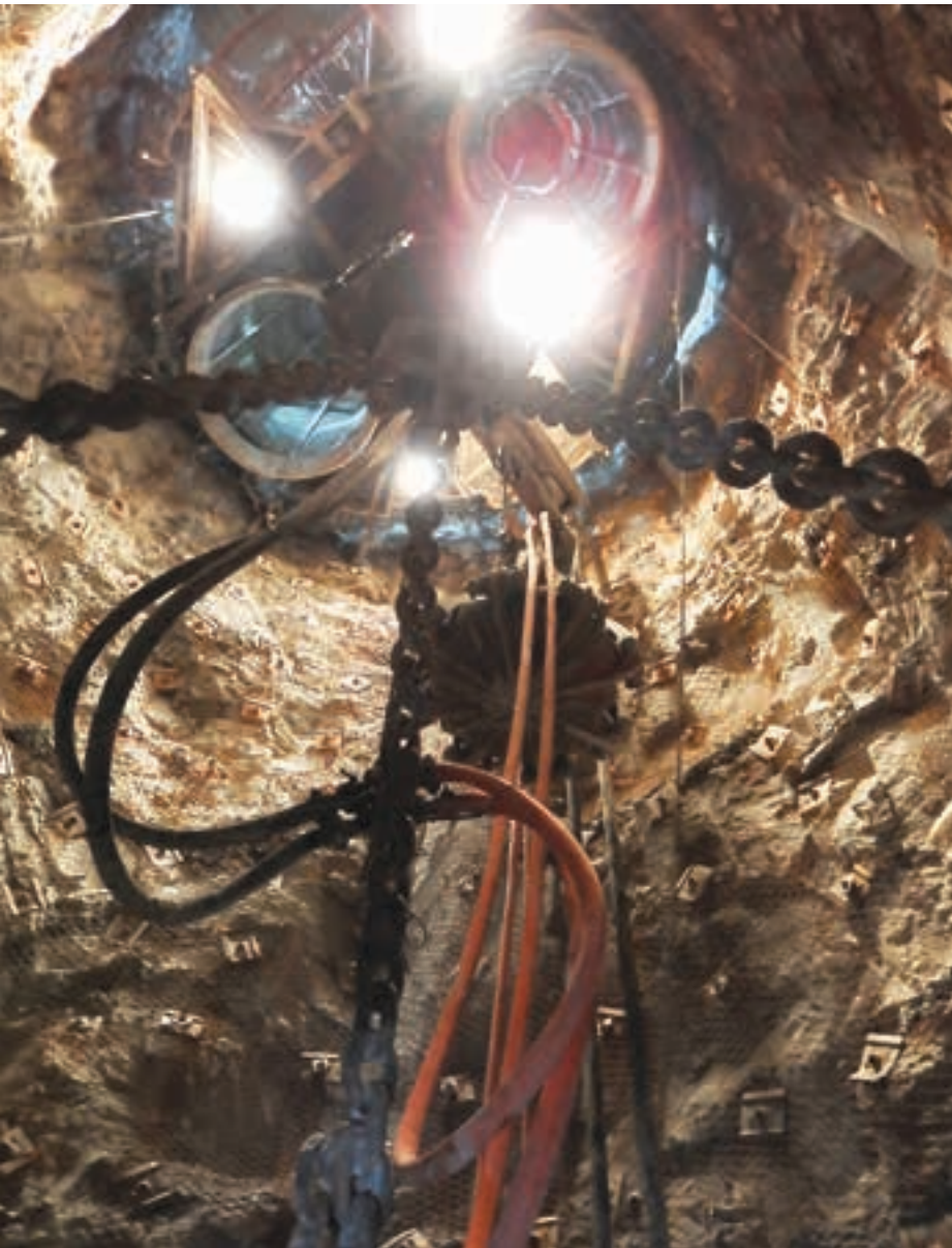
Looking up the ventilation shaft from the kibble towards the sinking stage (photo: Arthur Tassell).
