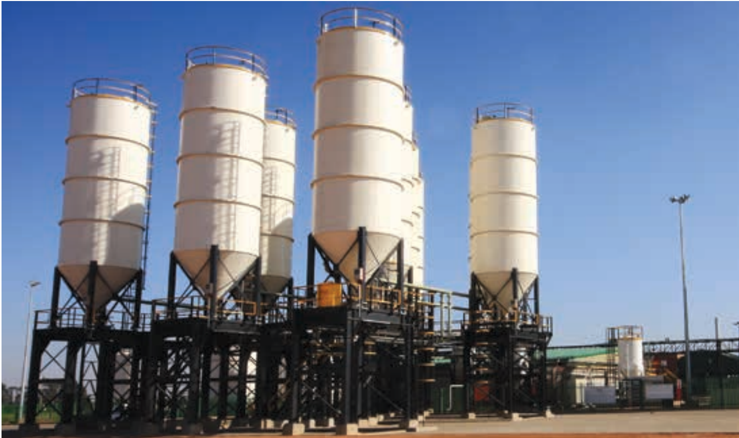
BME's emulsion plant at Dryden showing hot solution tanks and finished product silos.
