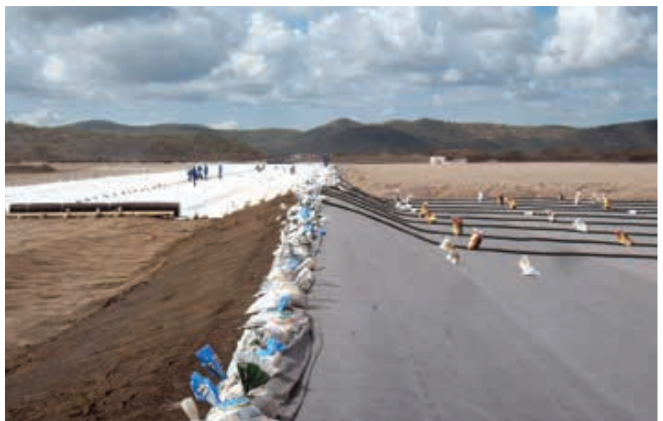
Heap leach pad construction at Tschudi in November last year.
