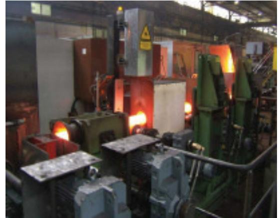
Inductive heating plant with a capacity of 2 x 1,800kW for reheating shells (Rohrwerk Maxhütte photo)
