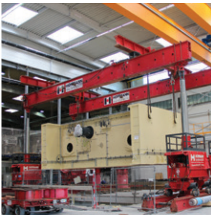
Lifting gear is used to add each component
