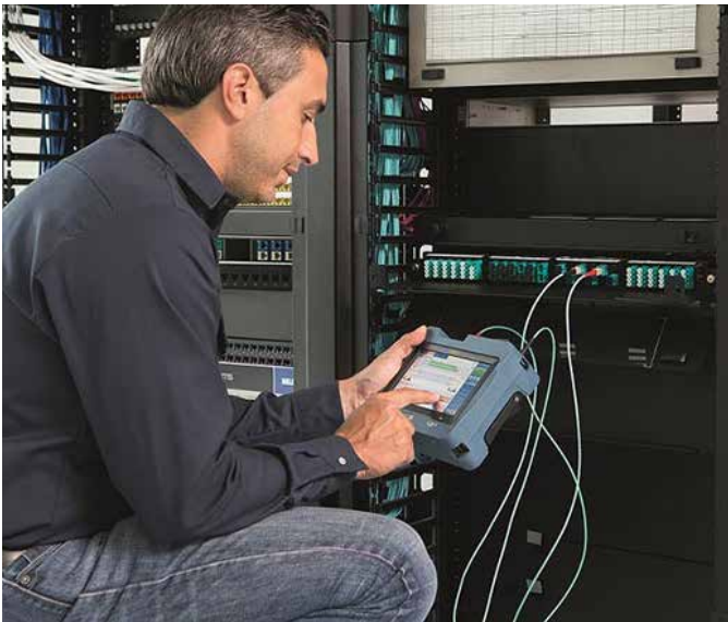
▲ The Optical Certifier I (OCI) for multi-mode and single-mode fiber cabling from Ideal Networks
