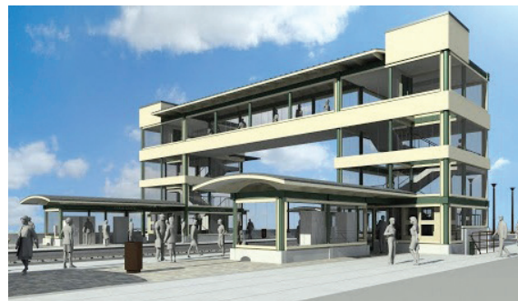
Example of two at-grade side platforms with shelters as well as elevators and stairs connecting to an overhead structure (roadway or pedestrian bridge)
