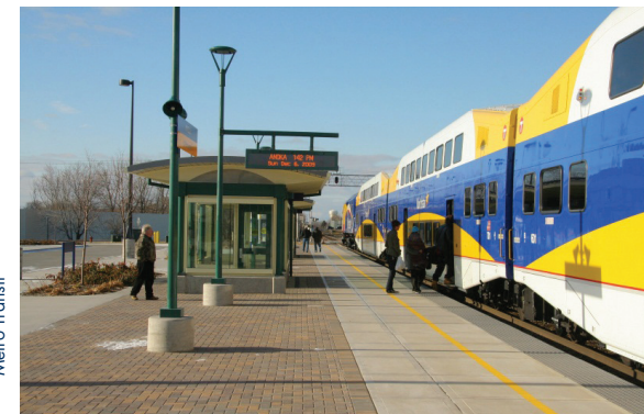
Example of at-grade station platforms with shelters
