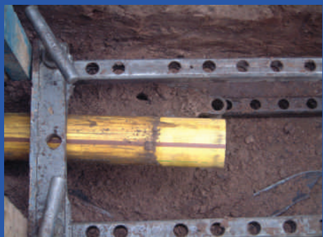
▲ Pipebursting with Uponor's ProFuse 110mm pipe
