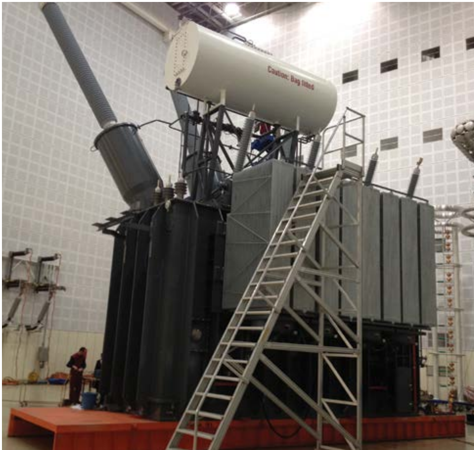
Figure 1: Transformer being tested at the factory.
