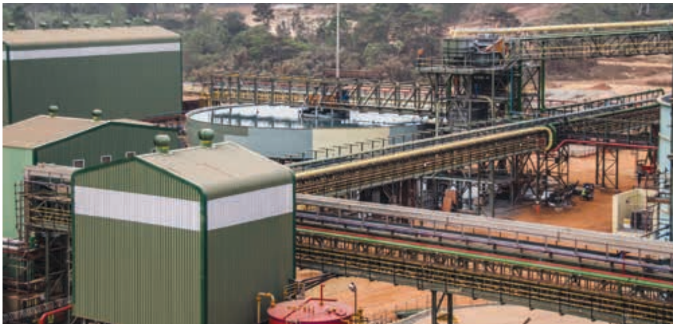
The Asanko plant area showing the pre-leach thickener (photo: Asanko Gold).
