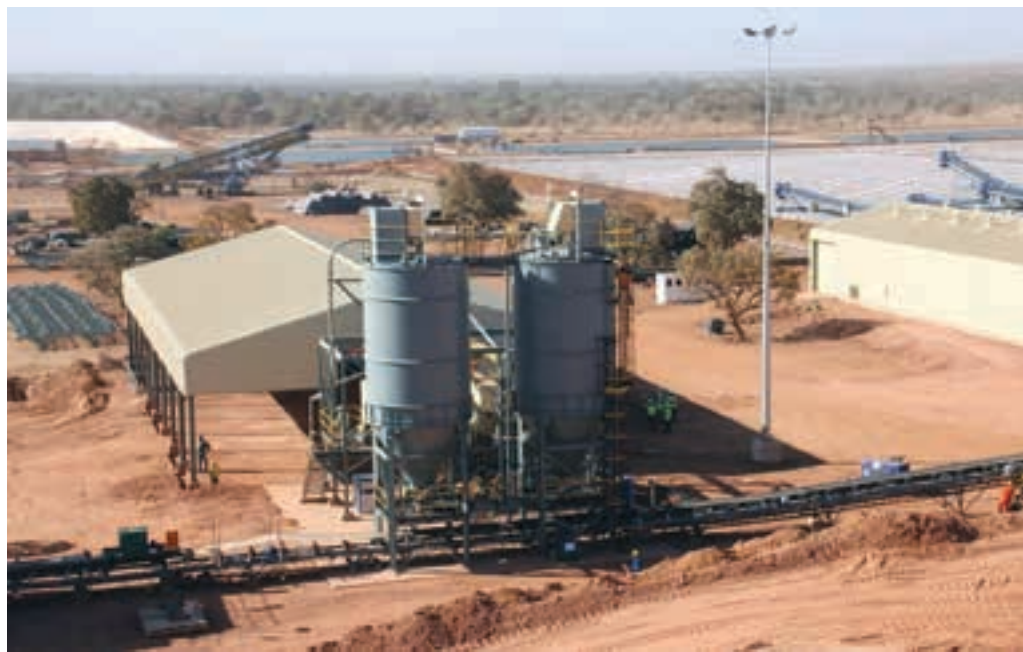
A recent view of the Karma site with cement silos in the foreground (photo: True Gold).
